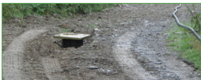
Position of first bleed valve for ridding the system of air locks
