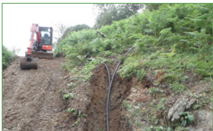
New track through the woods to the new tanks, showing old (thinner) and new (thicker) pipework
