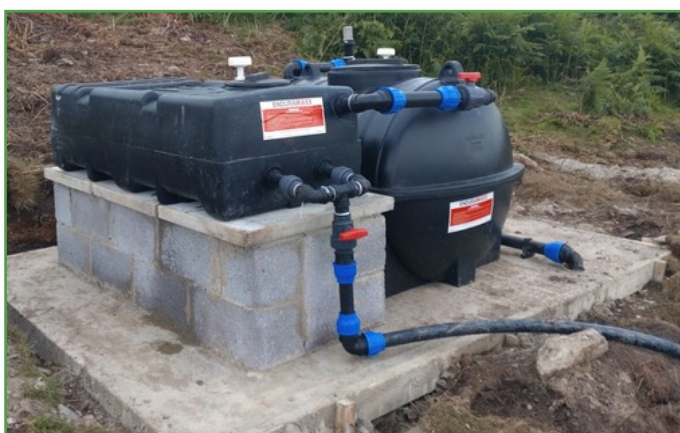
Foundation being constructed for settlement tanks
