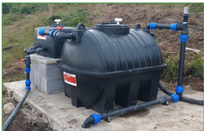
New settlement tanks plumbed in
