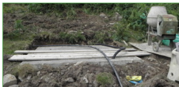
Foundation being constructed for settlement tanks
