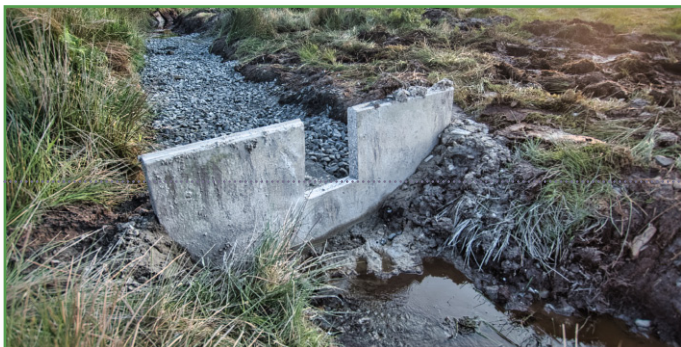
Dam constructed and trench filled with limestone chippings
