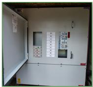
The final solution to this was to separate the properties from one major supply and create two separate supplies. This took six electricians a whole day and a new armoured cable as the old cable originally installed in 1979 had corroded and this was causing the fuses to blow it also required two new circuit boxes as the old ones were not fit for purpose. It was all put right on the 30/03/2023.
